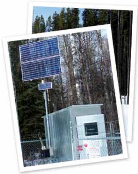
*GPT offers a line of Hybrid systems, combining solar with generators, and can convert any solar system to a hybrid with a thermoelectric or other type of generator.*
